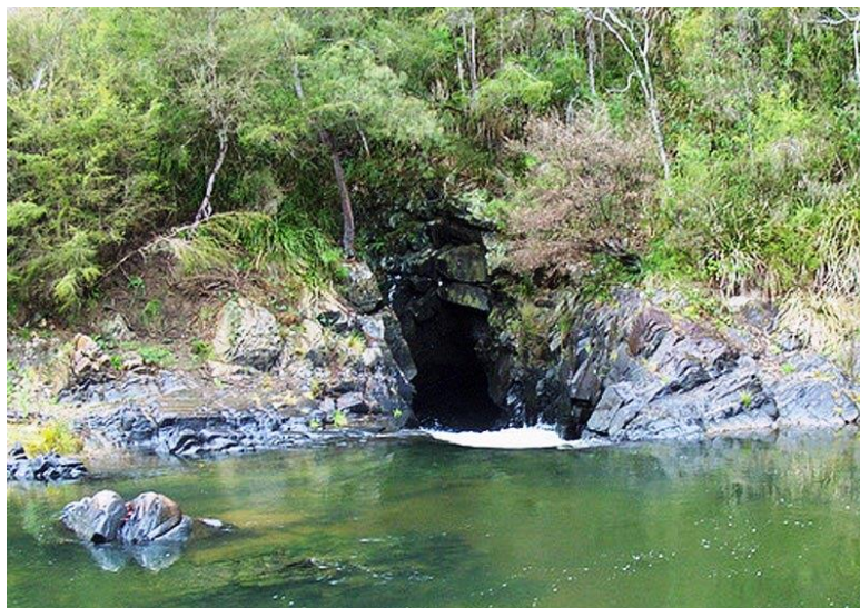
Horseshoe Bend Tunnel - Inlet
