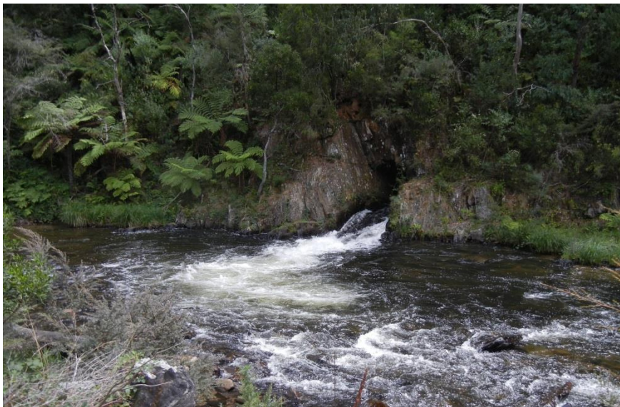
Horseshoe Bend Tunnel - Outlet
